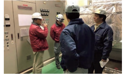
Energy Saving Diagnostics
