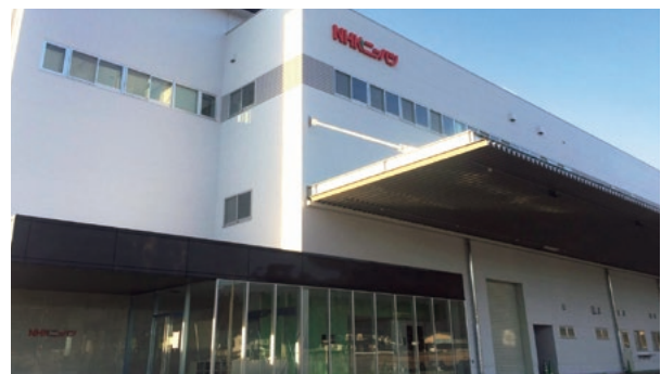
Completed Building at Miyada Plant
