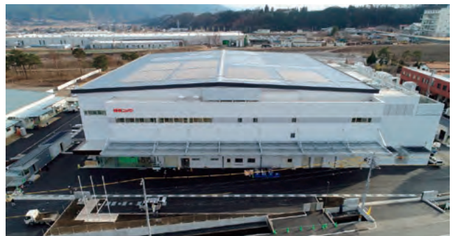
Miyada Plant (144kW, FY2018 operation start)
