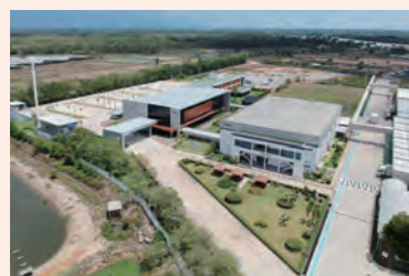
The Training Building is equipped with seven "Dou-jo"s (study rooms) to study the knowledge and skills that form the basis of production, such as safety, quality, and TPS.
