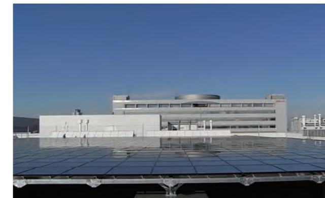
Yokohama Office (100kW, Start from FY2009)
